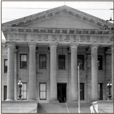
Fifth Street Entrance
